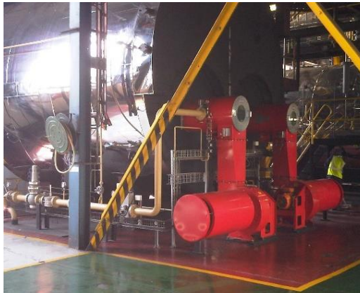
Installed Limpsfield LC200 (top), and 2 OFF LC88 (bottom) burners at SAB Rosslyn, South Africa, Photographs courtesy of Combustion Technology Ltd.
