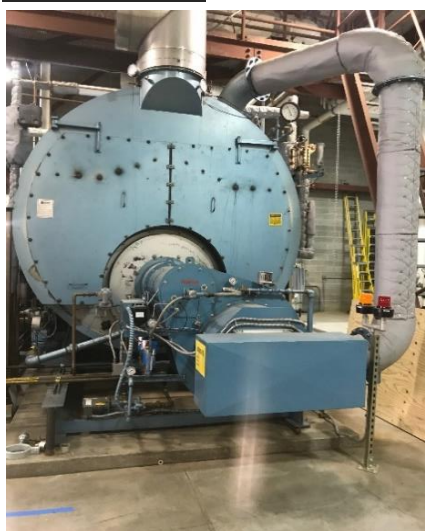
Before (left) and After (right) the installation and commissioning of the Limpsfield LC100 Burner on Superior Boilers. Photograph courtesy of Macdonald Miller.
