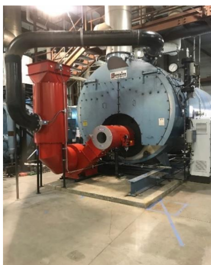
Before (left) and After (right) the installation and commissioning of the Limpsfield LC100 Burner on Superior Boilers. Photograph courtesy of Macdonald Miller.
