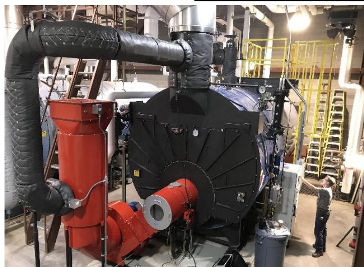
Limpsfield LC100 Burner on the New Hurst Boiler. Photograph courtesy of Macdonald Miller.
