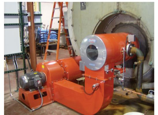
On completion of the install Wincup immediately saw great fuel savings of 12% with the burner running extremely efficiently at less than 3% O2 throughout the firing range, 0ppm CO and less than 10% CO2. As well as great fuel savings Wincup were also impressed with the reliability the Limpsfield burner produces.
